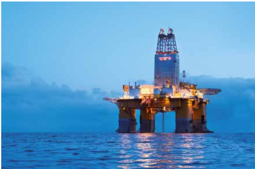
Fig. 3.8 Odfjell deep-sea offshore drilling rig in the Atlantic.
